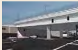
LRT maintenance yard at Valley Blvd.
